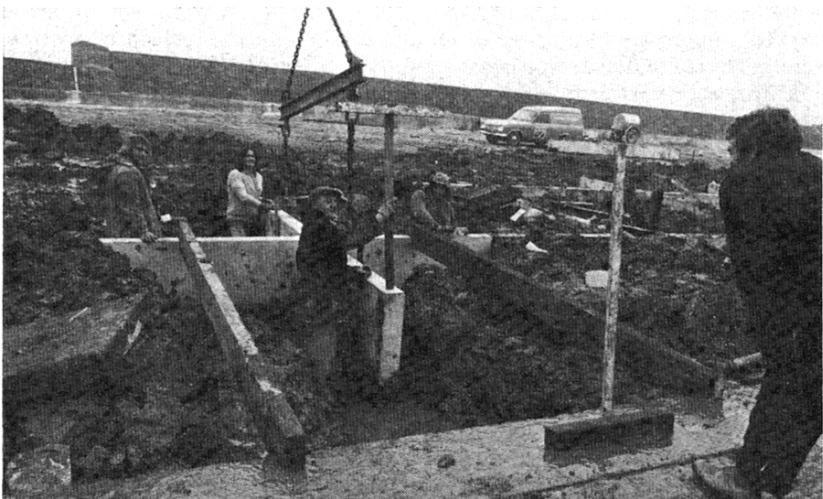
Fig. 14. Placing precast cruciform units in stage I facing
