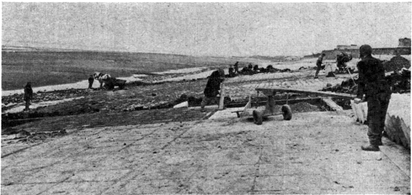
Fig. 8. Cellular paving under construction by manual method, 1949
