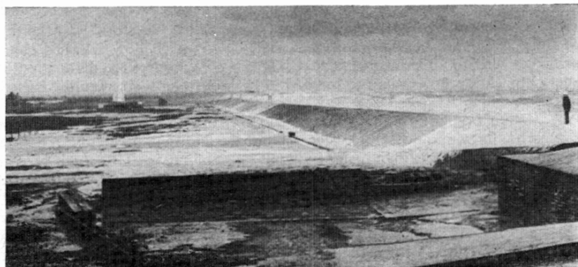
Fig. 6. Overtopping of embankment during NW gale, 2 April, 1973
