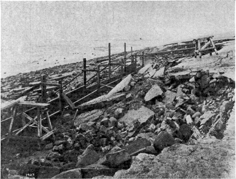
Fig. 7. Storm damage incurred during December 1919 showing cut-offs walls under construction
